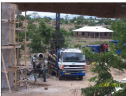
Drilling the borehole, completed February 2011
