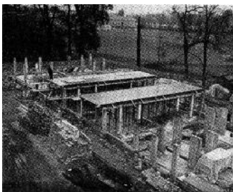
The Library and Chapel under construction in 1962.
