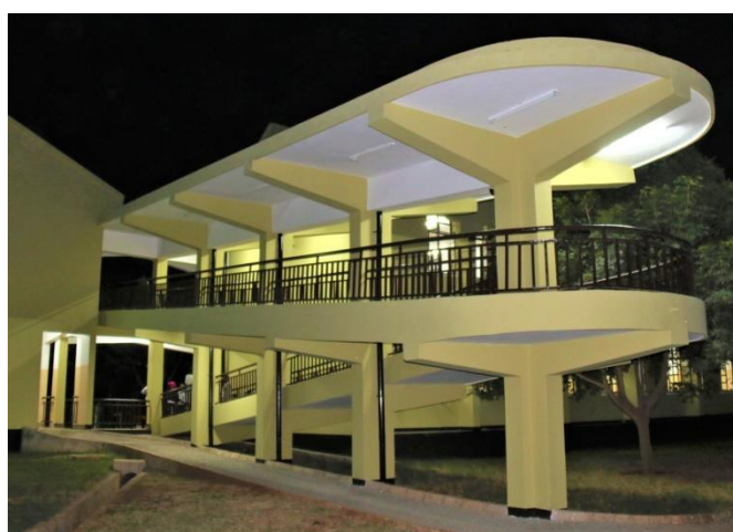
One of the disabled ramps fully lit by solar power as it climbs to the second-floor classrooms
