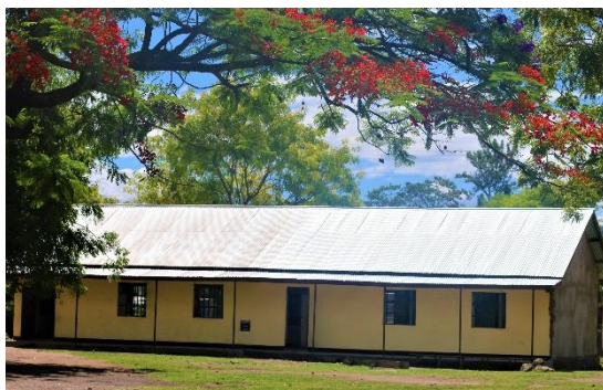
The new classroom at St Jude Thaddeus primary school. It has been linked with the classroom constructed in 2018.
