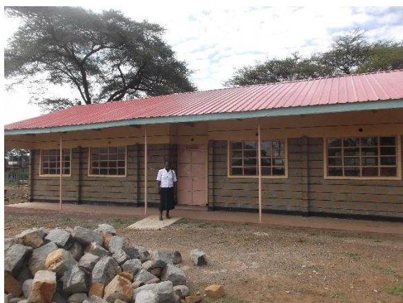
Sister Florence Boyani stands in front of the new classroom at St Paul's primary school.
