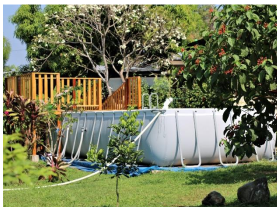
The hospice hydrotherapy pool. The ramp and seating area can be seen in the background.
