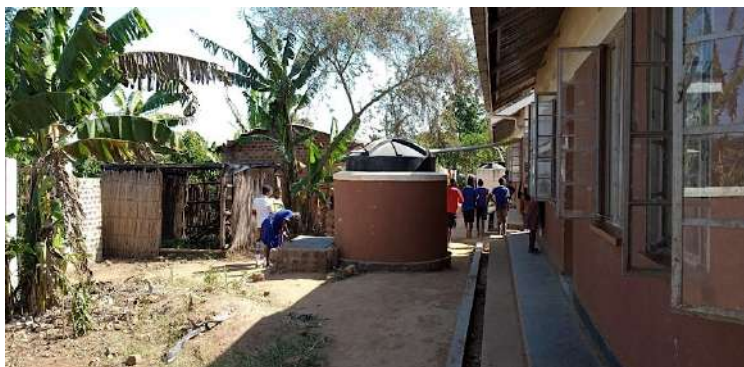
A 20,000 litre ferro-concrete water tank will be constructed at St Jude's, Masaka. It harvests water from the classroom roof.
